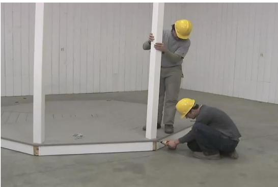
**Step 4:** Fasten posts to the floor with one 10 x 3 S.S. screw at each corner. Use only one screw to fasten posts until rails are fastened.
