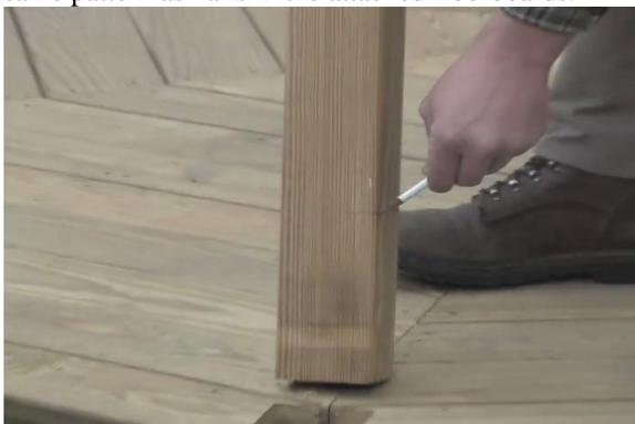
**Step 4:** Posts have a pencil mark that should be at the surface of the decking
